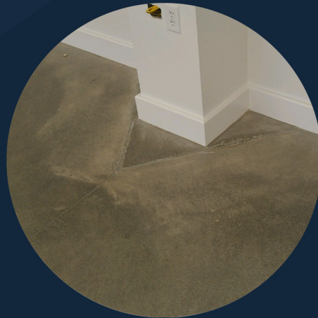
Variation from concrete finishing
